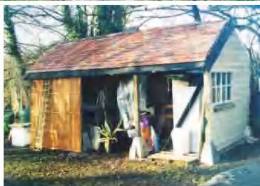
PIC 1. (RIGHT): The basic shed structure before the garden developed. This shed is now 16-years-old and the posts are still sound
